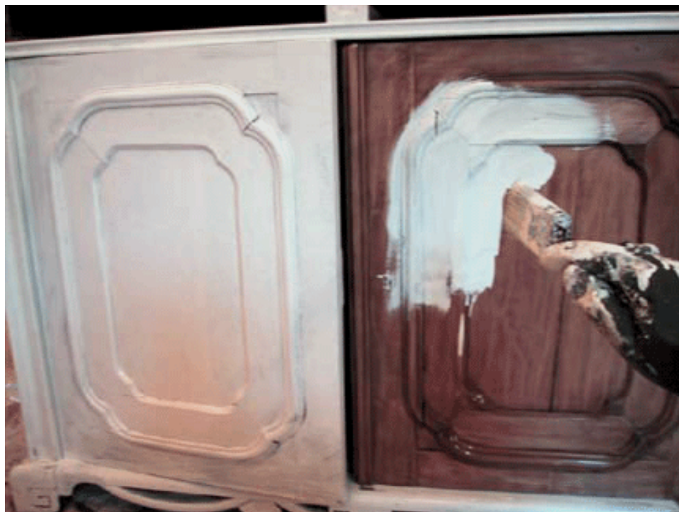
Priming the cabinet with a high quality, white primer.
