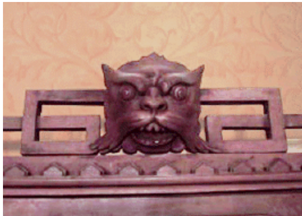
An un-finished detail.
