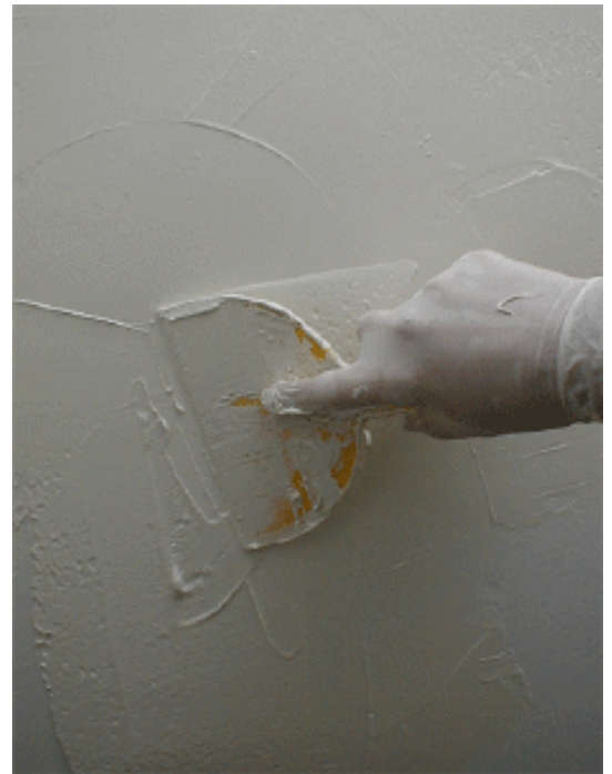
Wipe the trowel blade against another putty knife frequently to remove excess plaster build up.
