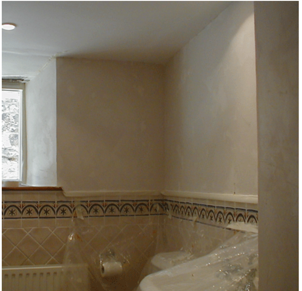
Completed plaster surface
