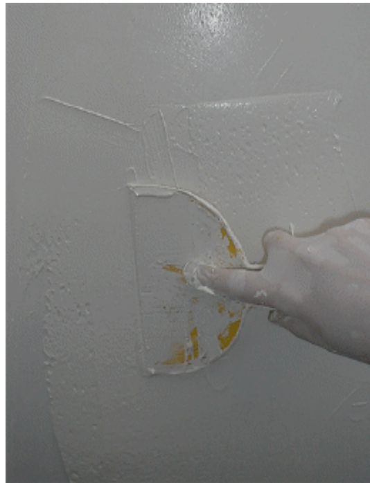
Carefully re-work the plaster to smooth and create light texture.
