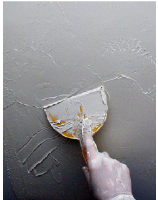
Creating a slight texture is an important part of the antique fresco appearance.
