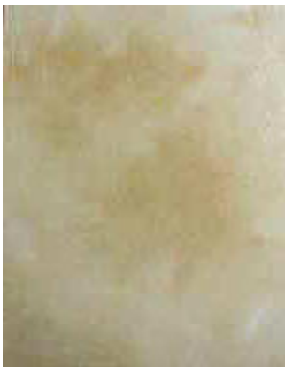
Detail of color washed wall surface.
